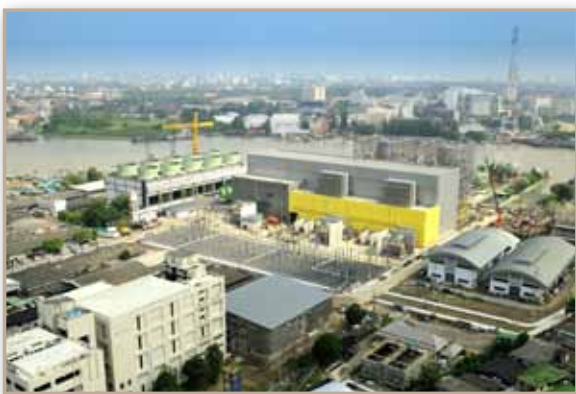
North Bangkok Combined Cycle Power Plant Block 2
