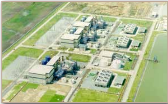
Wang Noi Combined Cycle Power Plant Block 4
